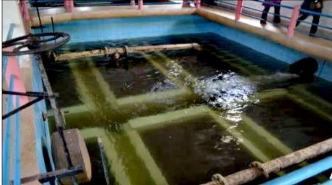
Fig.3.3. Sand filtration bed
